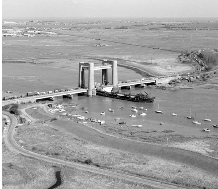
Instant traffic queues caused by the lifting of the bridge
