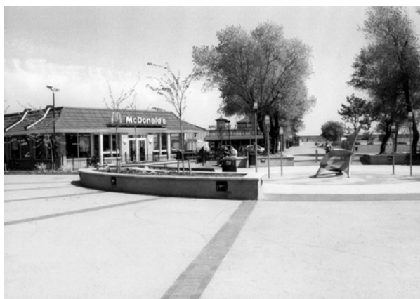
The Island's only McDonald's Restaurant – completed in 2000
