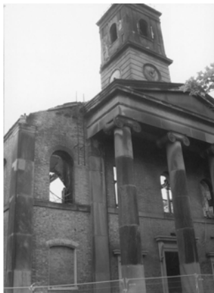
The Dockyard Church – in need of restoration
